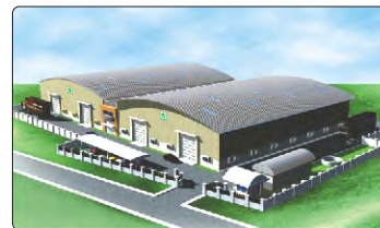
VANJAX FACTORY UNIT -2 (VXC-2)
